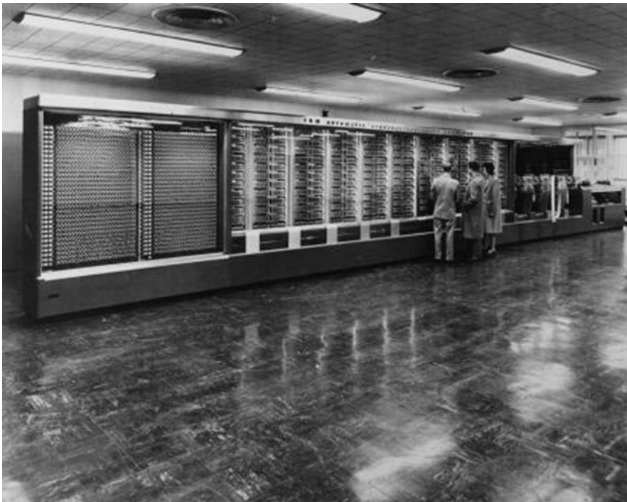
Figure 1-7 The Aiken/IBM Mark 1 Computer installed at Harvard, photograph IBM Corporate Archives.
